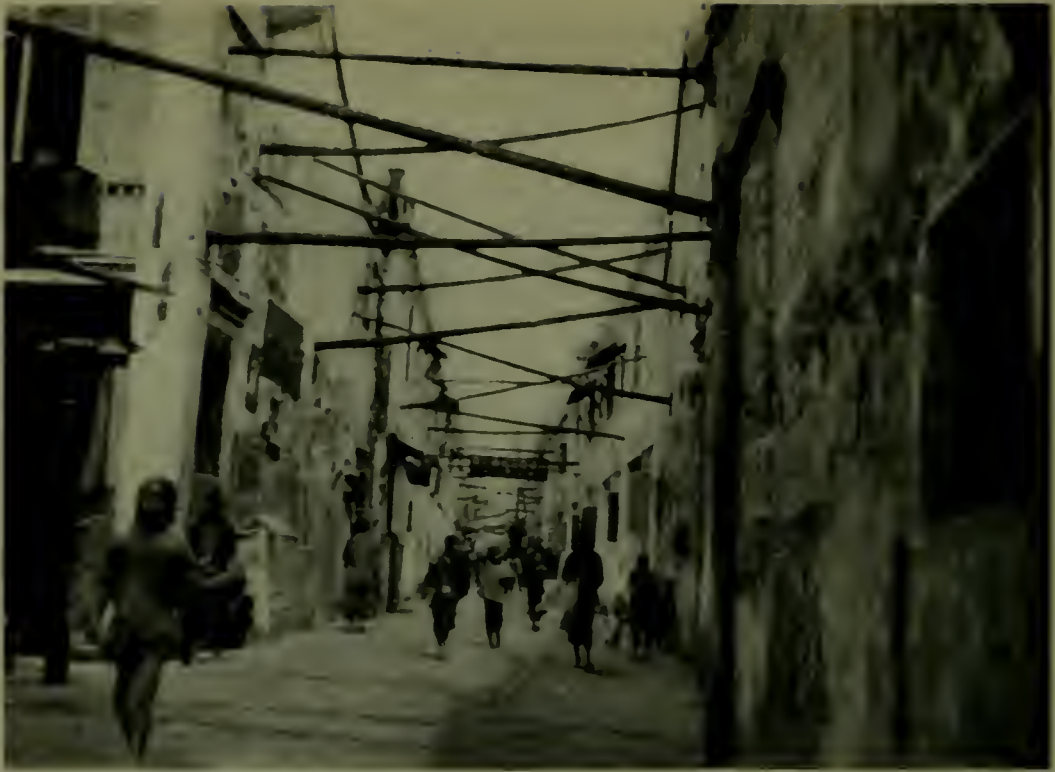
The typhoon and tidal wave that struck Swatow not only wiped out many houses and thousands of people but left whole streets so shaky that braces across them are necessary
